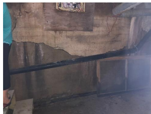
Figure 2.6: Curling Rink Basement Wall
