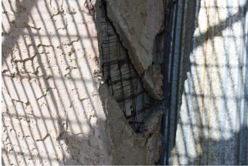
Photograph 15: Exterior finishes on the south portion of the Curling Rink (June 23, 2021).
