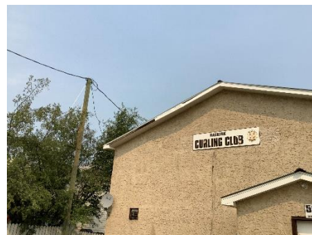
Figure 2.5: Curling Rink Exterior
