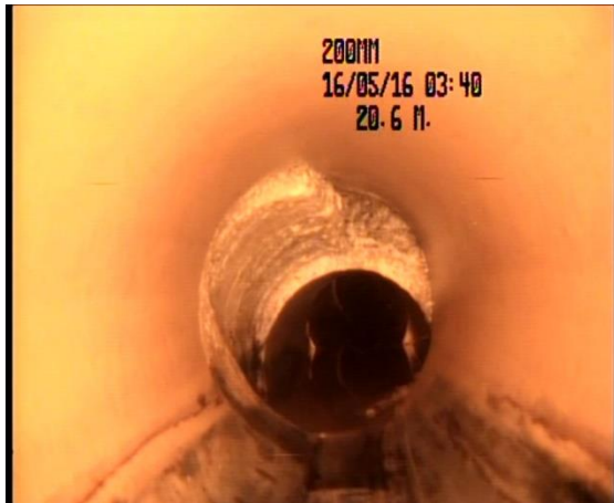
Figure 3.4: Severe Offset
