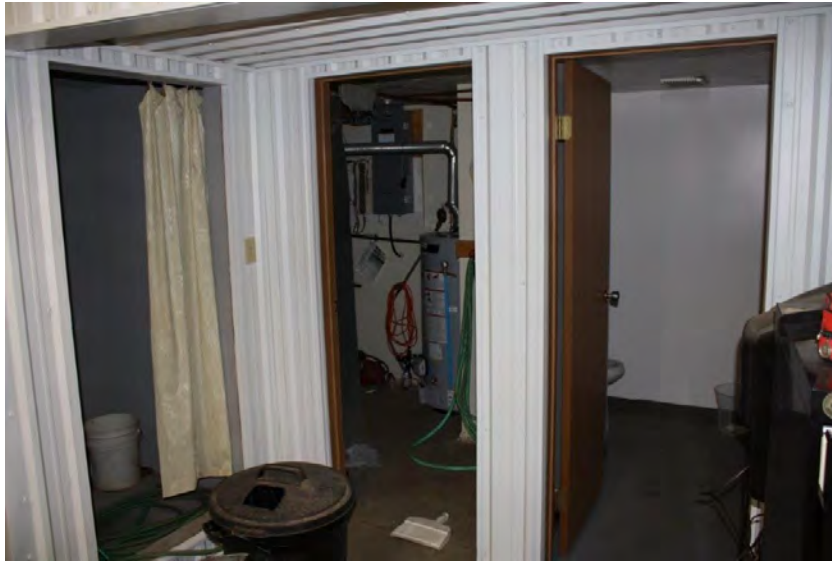
Photograph 41: The showers, mechanical room and lunch room under the mezzanine in the Fire Hall (June 23, 2021).
