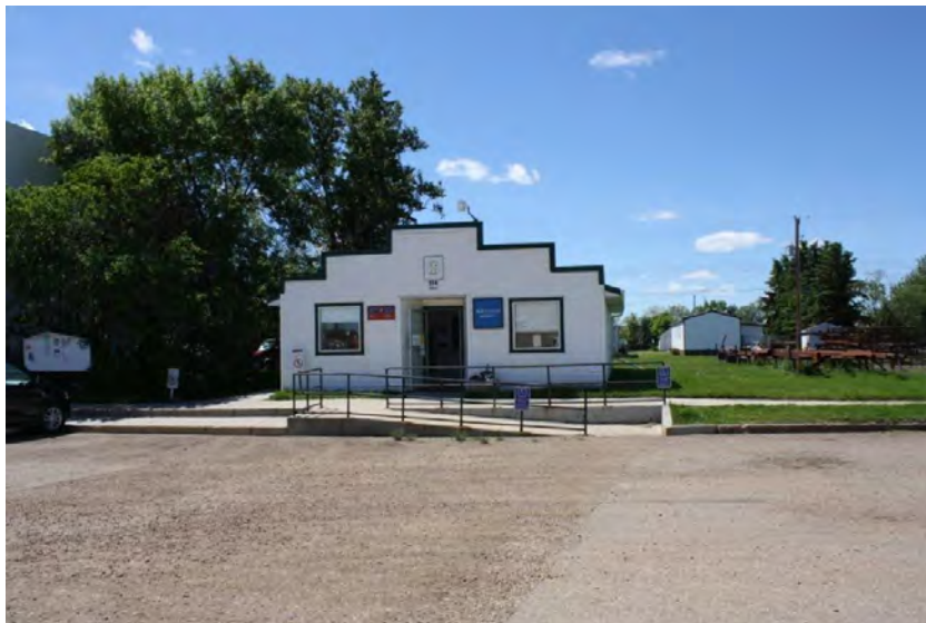
Photograph 44: Looking west across Main Street towards the Canada Post and Bank building (June 23, 2021).
