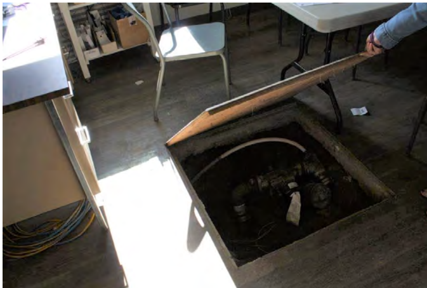
Photograph 42: The septic cleanout in the lunchroom in the Fire Hall (June 23, 2021).
