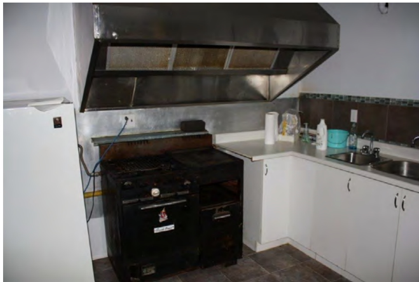
Photograph 6: The main floor kitchen in the Curling Rink (June 23, 2021).
