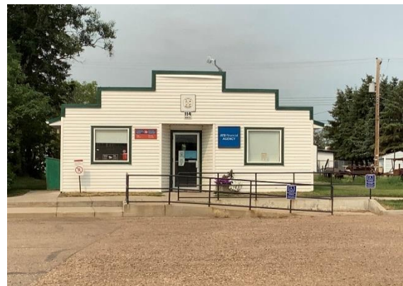
Figure 2.10: Canada Post Office Exterior
