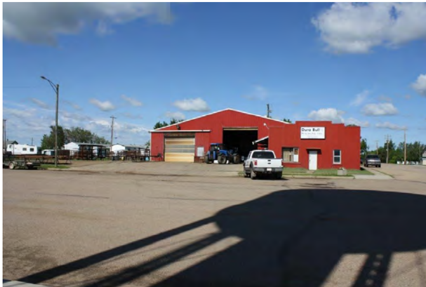
Photograph 5: Looking west across Main Street, south of Alberta Avenue at Dura Bull, a site with reported USTs in the 1960's (June 23, 2021).
