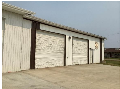
Figure 2.7: Fire Hall Exterior
