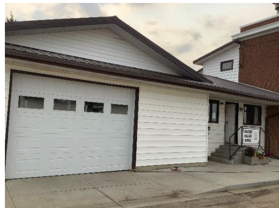
Figure 2.13: Village Office and Public Works Shop Exterior
