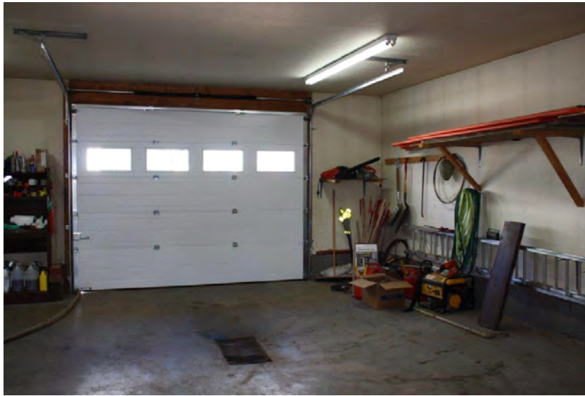
Photograph 17: The west portion of the Public Works shop (June 23, 2021).
