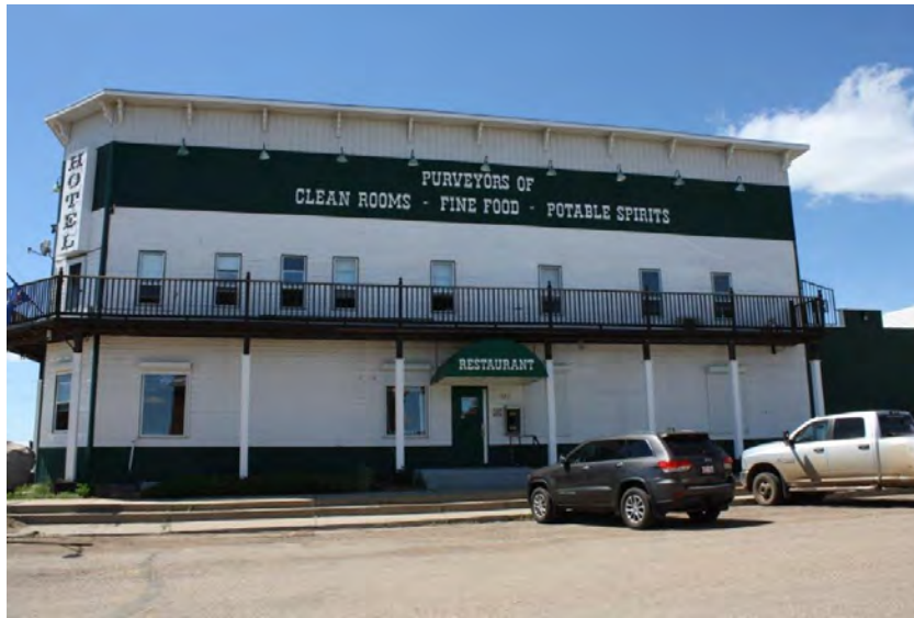
Photograph 1: Looking east at the Halkirk Hotel from Main Street (June 23, 2021).
