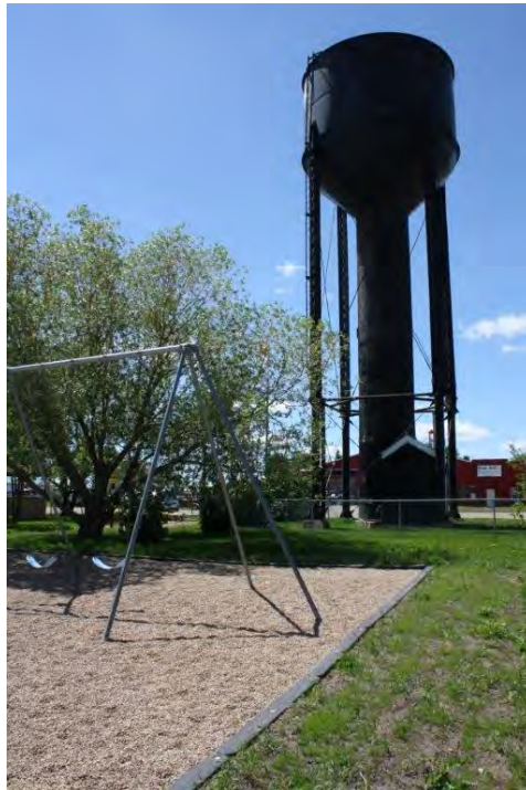
Photograph 33: Looking west across the north side of the Playground toward the Water tower (June 23, 2021).
