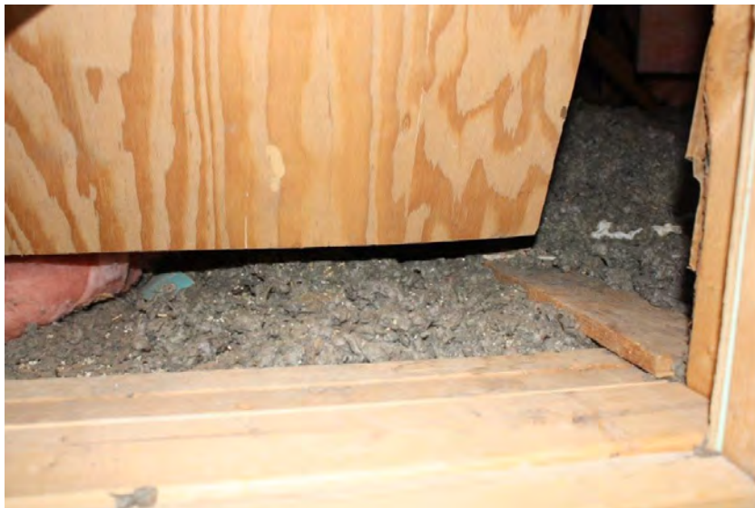
Photograph 30: Insulation in the attic of the Community Hall (June 23, 2021).
