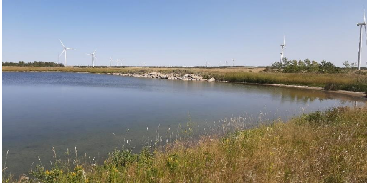
Figure 3.9: Recycled Concrete Erosion Protection
