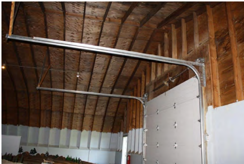
Photograph 6: The uninsulated ceiling and overhead door on the north portion of the Mini Arena (June 23, 2021).
